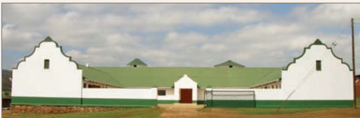
The newly renovated Opstal
